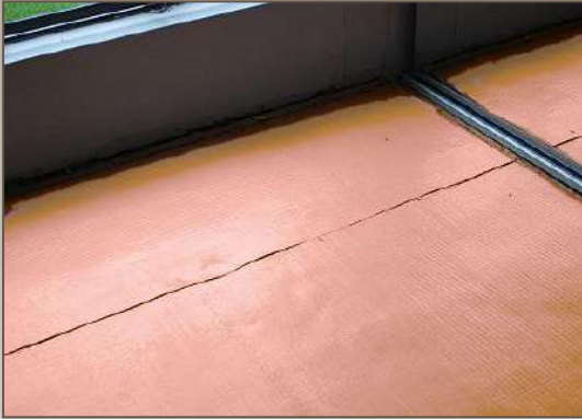
1. Underfelt or foam underlay is laid by carpet installers.
