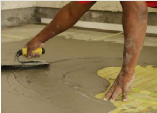
3. Protective screed is applied.
