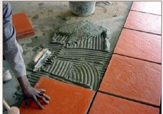
4. The floor is then tiled.
