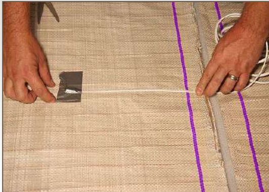
3. The probe for floor temperature limitation is placed and connected.
