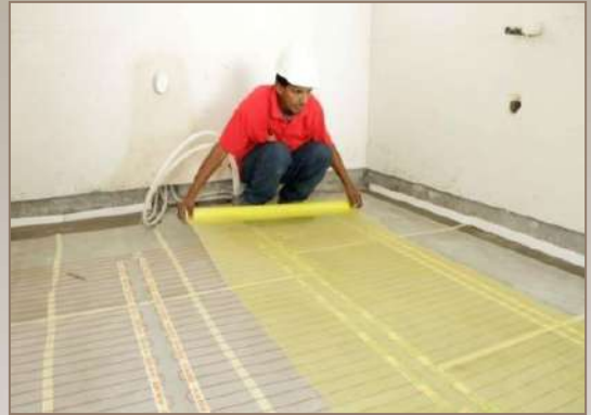
2. Adhesive mesh is then laid on top of the heating element
