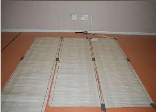
3. The carpet heater is secured down with tape.
